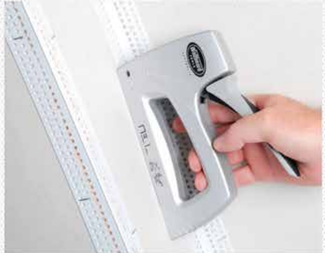
4. Staple through the mud leg at 200mm centres maximum using 10mm staples
