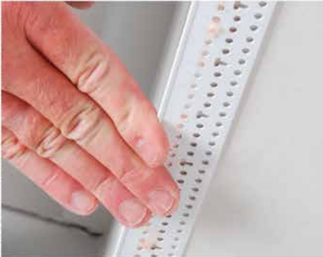
3. Apply firm, even pressure to the mud legs of the trim to ensure a solid bond
